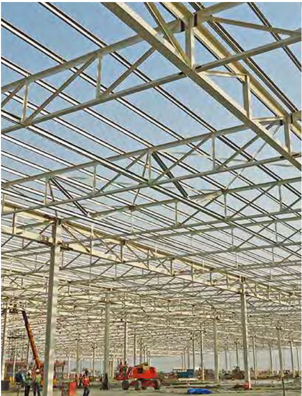
FORD (BY L&T LIMITED) Automobile Assembly Unit Roof Structure
